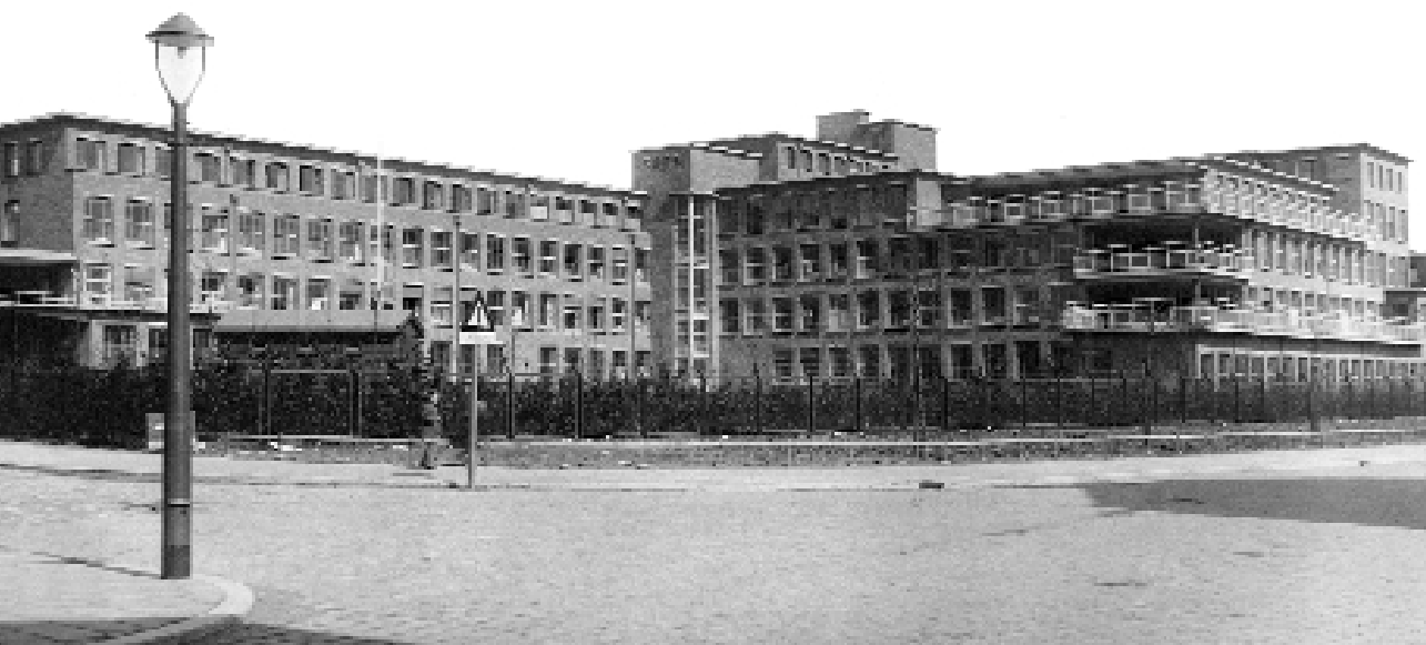
The new hospital complex shortly after completion. Top: Gordelweg façade with main entrance; bottom: back-front of the Children's Hospital, with left the neonatal unit and right the department of pediatrics, surgical department and service rooms.
